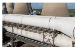
Safety concerns arise when the large fan blades need to be replaced per maintenance schedules. The blades are accessible through a hatch in the horizontal fan duct. As blades are removed, the assembly becomes out of balance, causing it to rotate. There is a small clearance between blade tip and duct and the inertia of the slowly rotating assembly makes it difficult to stop by hand. This condition presented a trap-risk for maintenance workers during the uncontrolled rotation.
